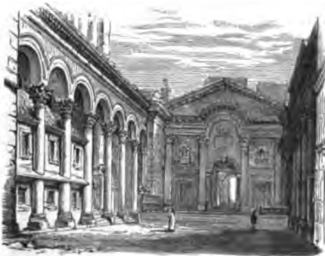
Fig. 2.—Courtyard at Spalato.
